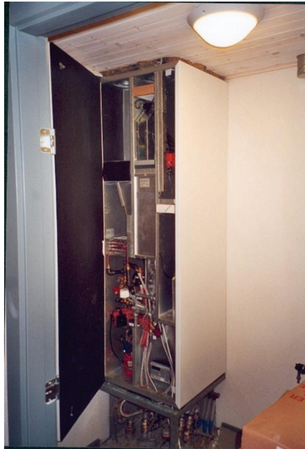
Figure 78: Cupboard with the combined solution of DHW supply and ventilation heating system.
