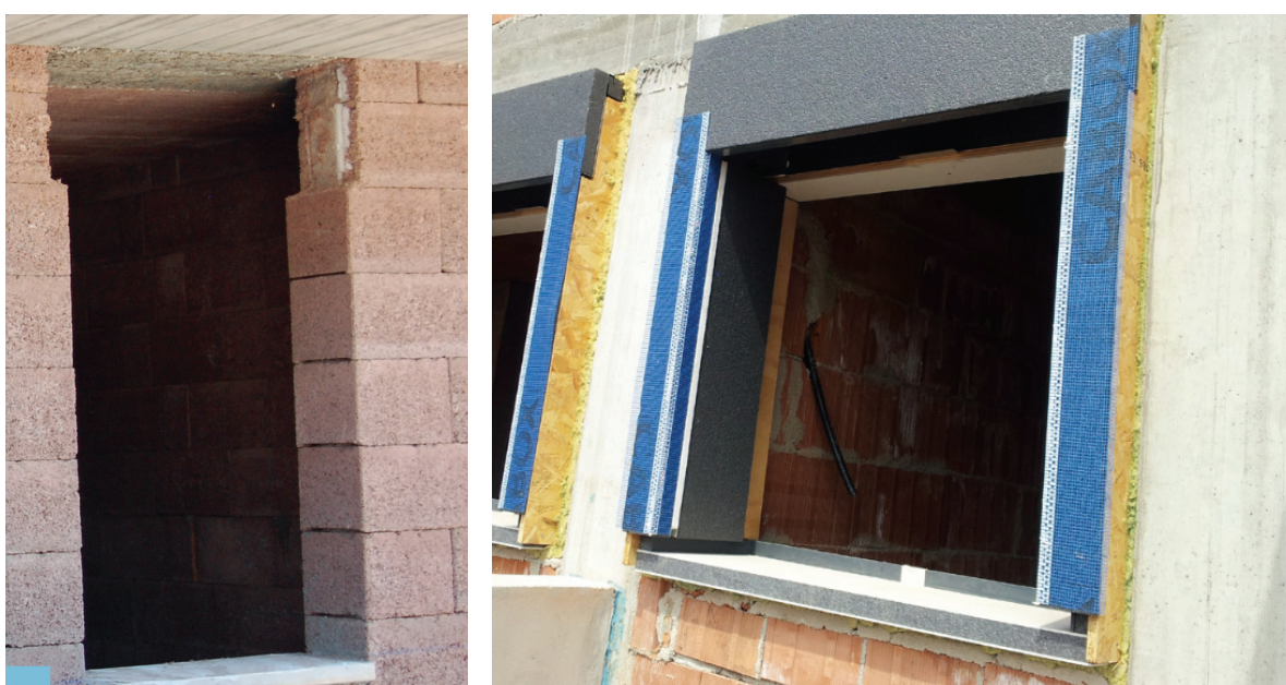
Figure 66: Example of mono-block window. Left the hole in the wall without subframe, right the window installed. Courtesy of Alpacom S.r.l.
