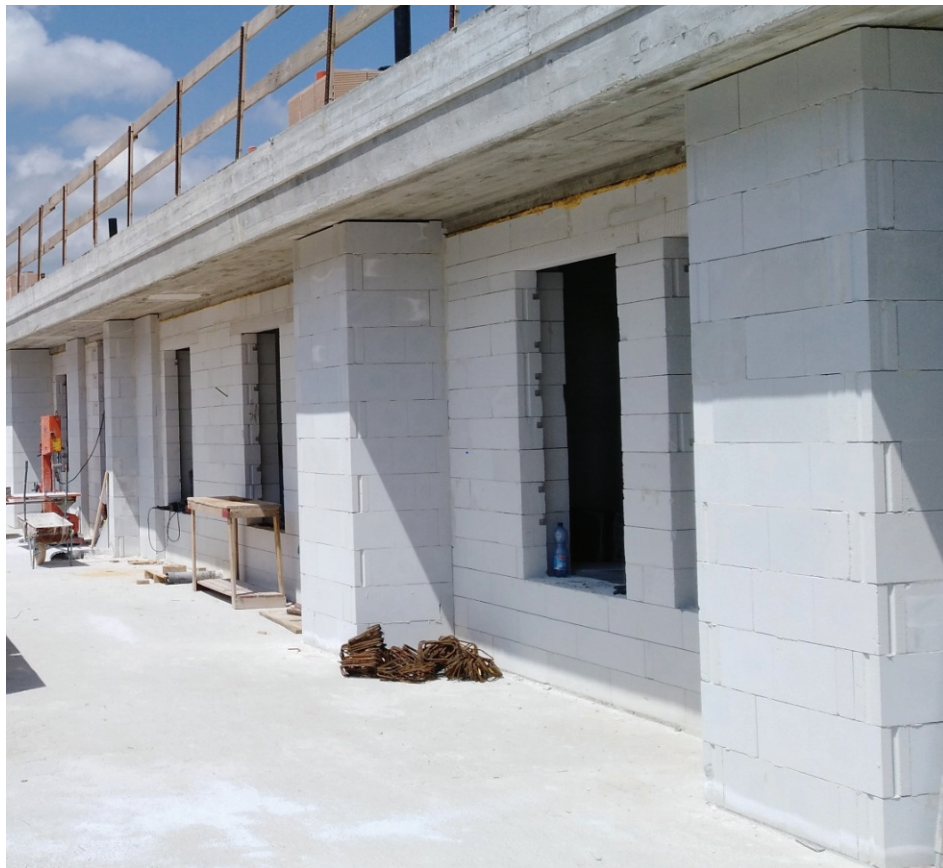
Figure 65: Example of construction works using autoclaved blocks. Courtesy of Xella Italia S.r.l.
