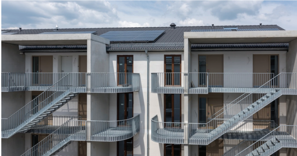
Figure 74: Photo of the external staircases of the Frankfurter Klimaschutzhaus. © Jochen Müller
