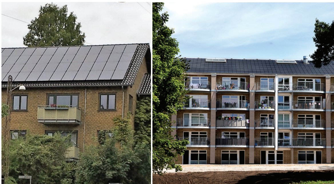
Figure 67: Buildings with conventional roof + PV (left) and PV integrated roof (right).
