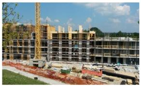
**Figure 7.** Construction phase – construction of the upper two floors in a wooden construction.
